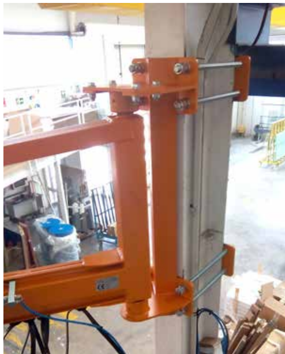
METAL COLUMN WELDING + REINFORCED BRACKETS
