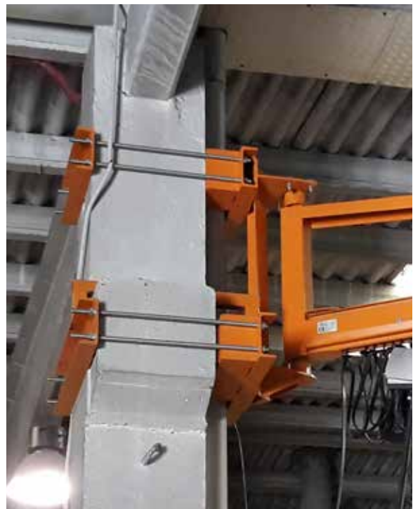
CONCRETE COLUMN BRACKETS
